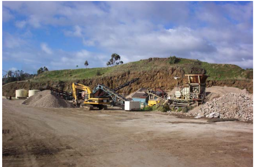
The concrete crushing plant at the Fyansford site
